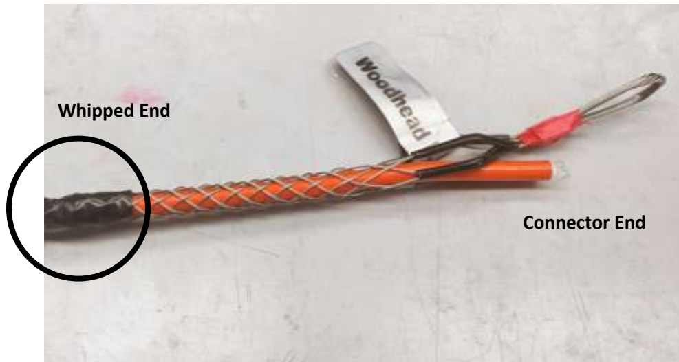
Figure 1: Applying electrical tape to cable grip and cable.
